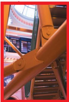
This is part of the steel structure which attaches the Theatre building to the columns. The columns support the 150 ton weight of the Theatre – without them it would fall through the floor into the shops underneath. If a big elephant weighs 6 tonnes, how many elephants would it take to match the Theatre's weight?
